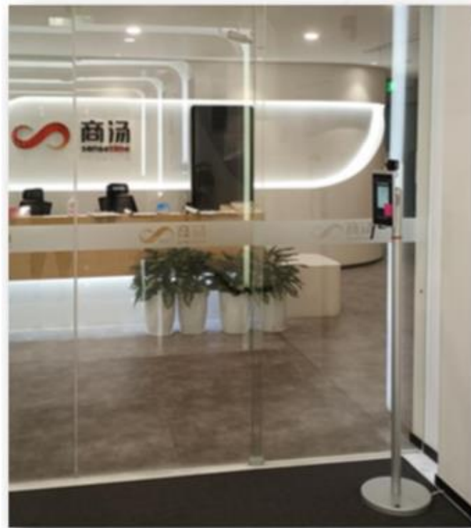
Vertical Stand installation
